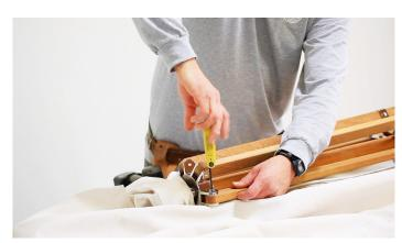
Replace the canopy by stretching the cover over the tips of the long arms, and into the pockets.
