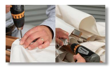
Re-attach the canopy with the screws and L-brackets that were removed, and re-attach the fabric straps from the main cover to the wind vent.
