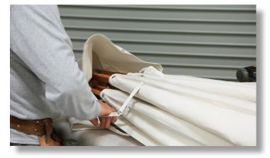
Partially remove the canopy, by removing the screws that attach it to the frame and the L-brackets.
