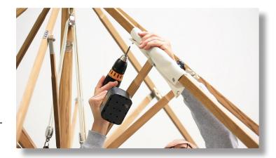
Slip the new cover over the frame, and attach it - first, at the ends of the arms with the L-clips, then at the top of the frame with the screws.
